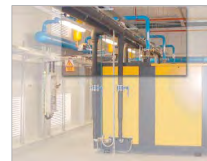
Fig. 3b: Vibration-dampening compressor connection with axial compensators
