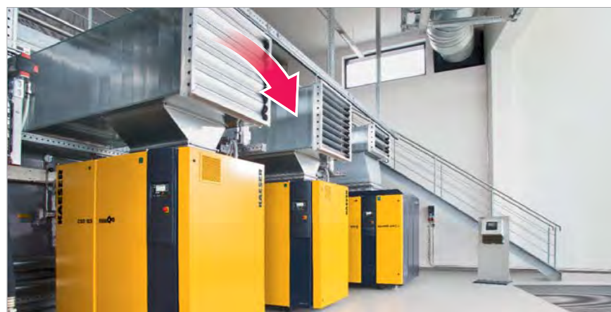
Fig. 3: Compressed air station with thermostatically-controlled air ducting
