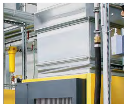
Fig. 2: Compressor ventilation connection with canvas duct joint
