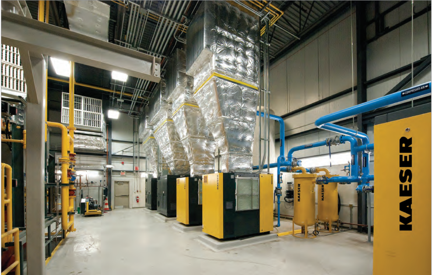
Heat from the new air compressors is recovered in the compressor area.
