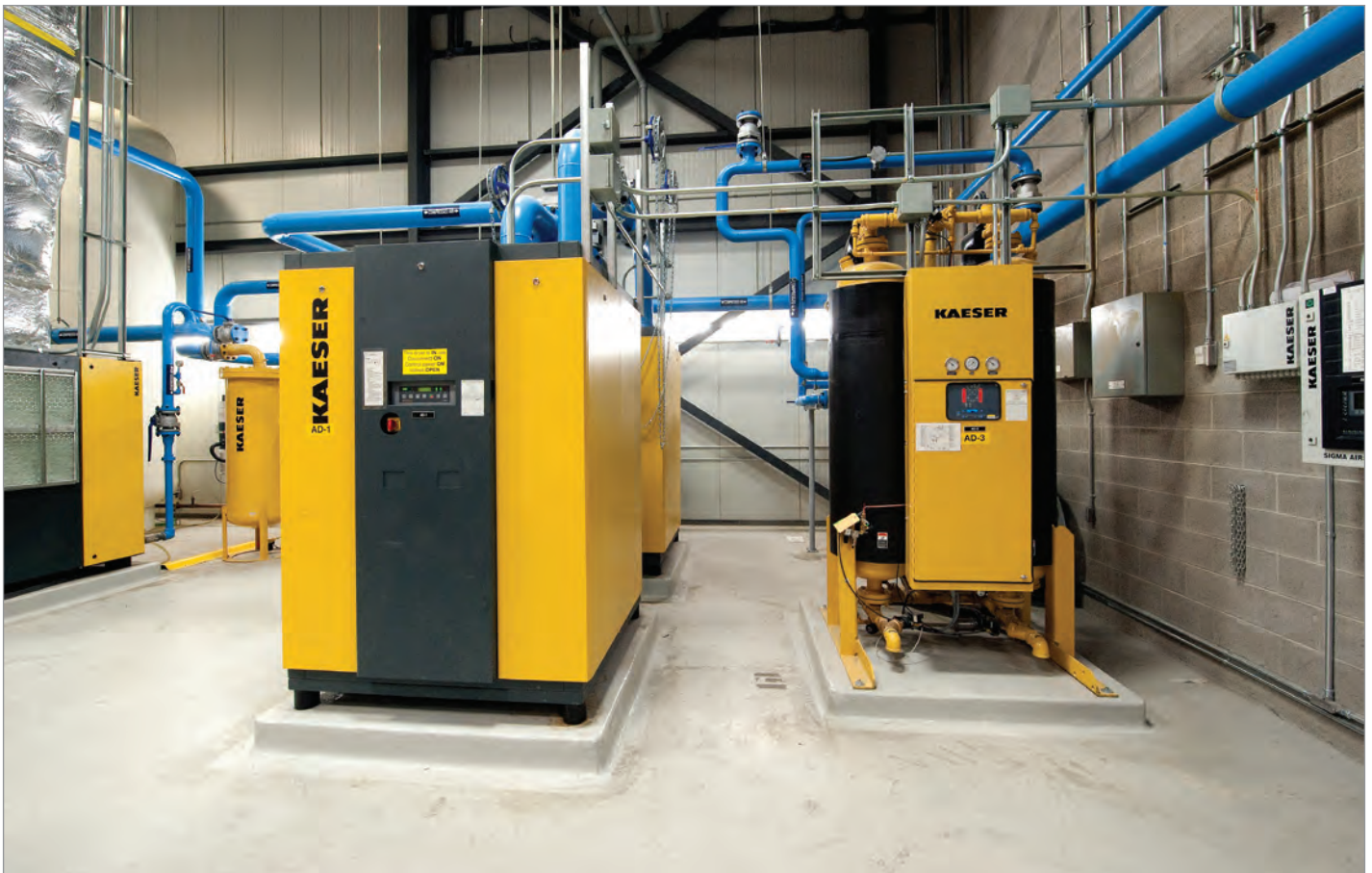
All compressors are controlled, within a narrow pressure band, by a sophisticated sequencing control system and the accurate regulation of the VSD compressors.
