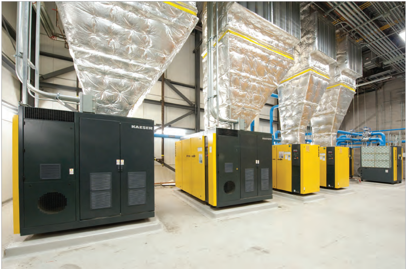
The new system uses four rotary screw compressors and two booster compressors.
